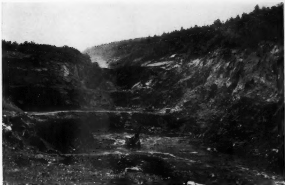
OPERATIONS IN THE LOWER PITS, BARTON MINES, NEAR NORTH CREEK, N.Y.
